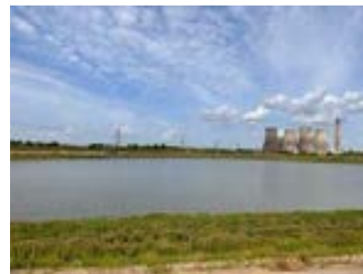
Picture 1: LAG1. Note the power station situated in the distance.
