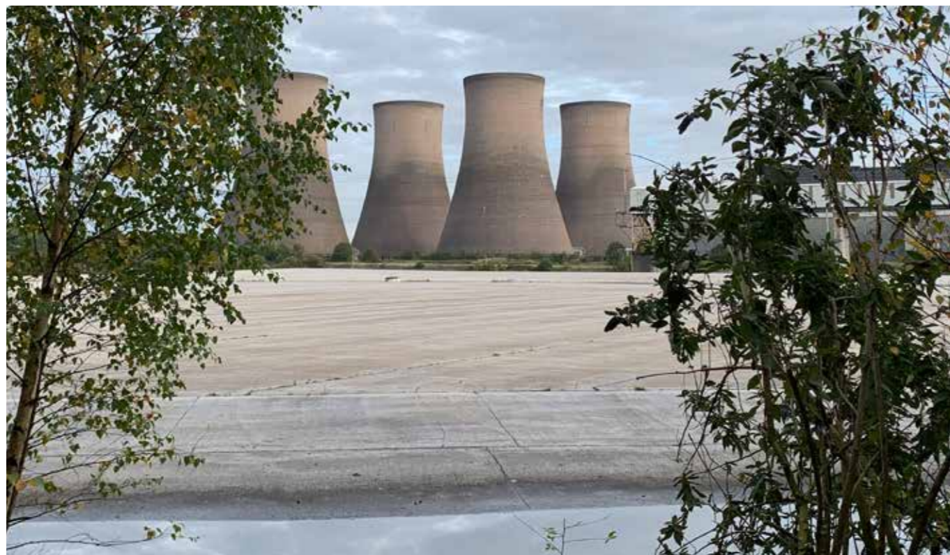
Looking east across the former coal stock yard
