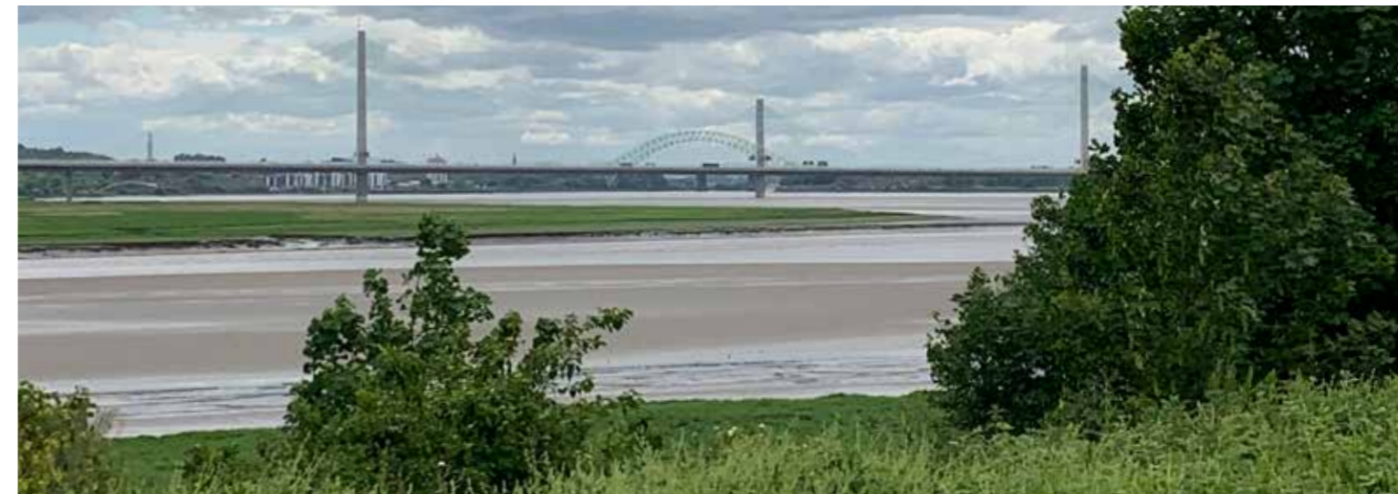
View out from the lagoon area towards the river foreshore and bridges
